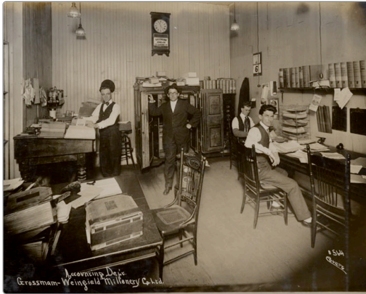
The Accounting Department of the Grossman-Weinfeld Millinery Company, New Orleans, Covert (photographer), 1917 · Photograph · New Orleans, Louisiana
