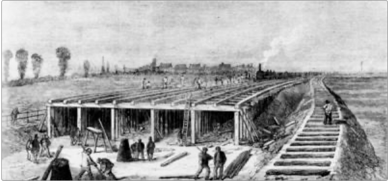
The Northern Outfall Sewer Under Construction , Illustrated London News, 1861 · Wood engraving · Published in London
