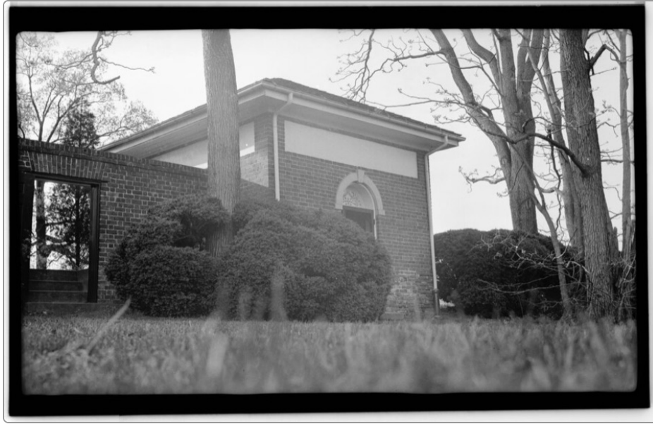
Smokehouse at Woodlawn, Fairfax County, Virginia , Historic American Buildings Survey photographer, 1930s · Photograph · Library of Congress, Washington, D.C.
