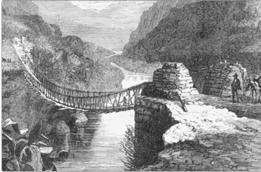
The Rope Bridge over the Apurímac River, E. George Squier, 1877 · Engraving · From Peru: Incidents of Travel and Exploration in the Land of the Incas
