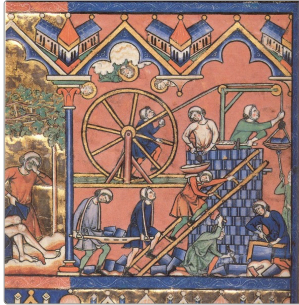
Building with a Treadwheel Crane , Unknown illuminator, 13th century · Manuscript painting (paint and gold on parchment) · A medieval French manuscript
