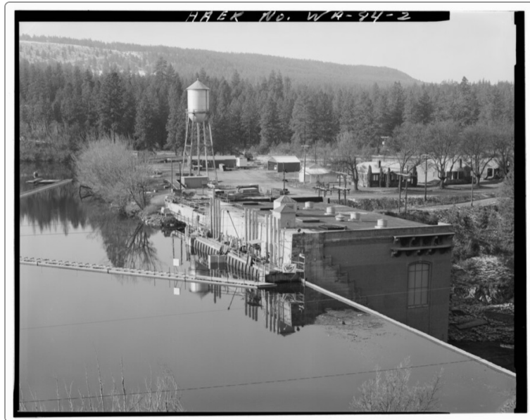
Nine Mile Dam and Powerhouse , Historic American Engineering Record, Powerhouse built 1908; photograph late 1900s · Photograph · Library of Congress, Prints and Photographs Division
