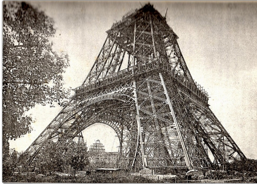
The Eiffel Tower Under Construction, July 1888 , From Louis Rousselet's book on the 1889 World's Fair, July 1888 · Photograph (printed in a book) · From L'Exposition universelle de 1889 by Louis Rousselet
