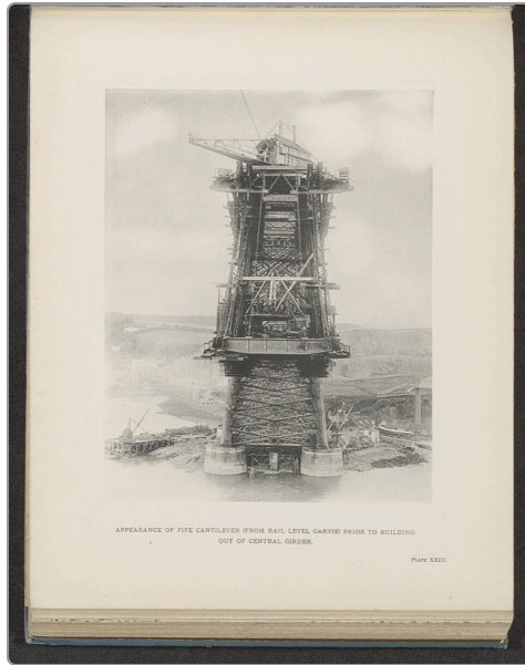
The Fife Cantilever Under Construction , Unknown photographer, about 1888 · Photograph · Rijksmuseum, Amsterdam
