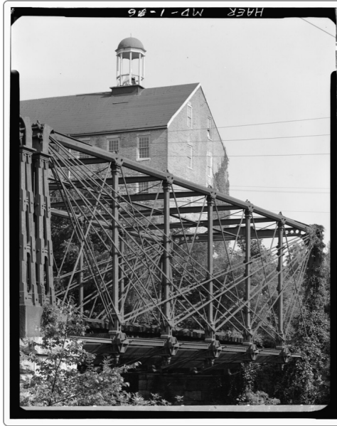
The Bollman Truss Bridge at Savage, Maryland, Historic American Engineering Record, Photograph of a bridge built in 1869 · Photograph · Library of Congress, Prints and Photographs Division
