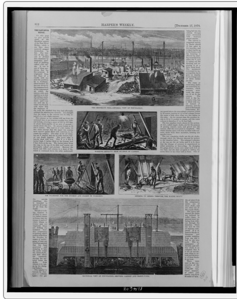
The East River Bridge: Inside the Caisson , Unknown engravers for Harper's Weekly , December 17, 1870 · Wood engravings in a weekly newspaper · Library of Congress, Prints and Photographs Division Image: Wikimedia Commons , public domain
