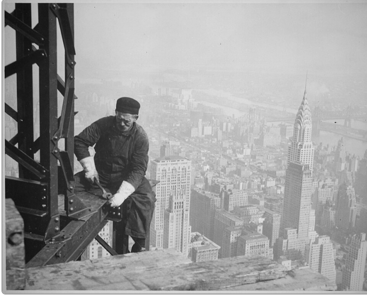
A Workman on the Framework of the Empire State Building , Lewis Hine, 1930–1931 · Photograph · National Archives, Washington, D.C.
