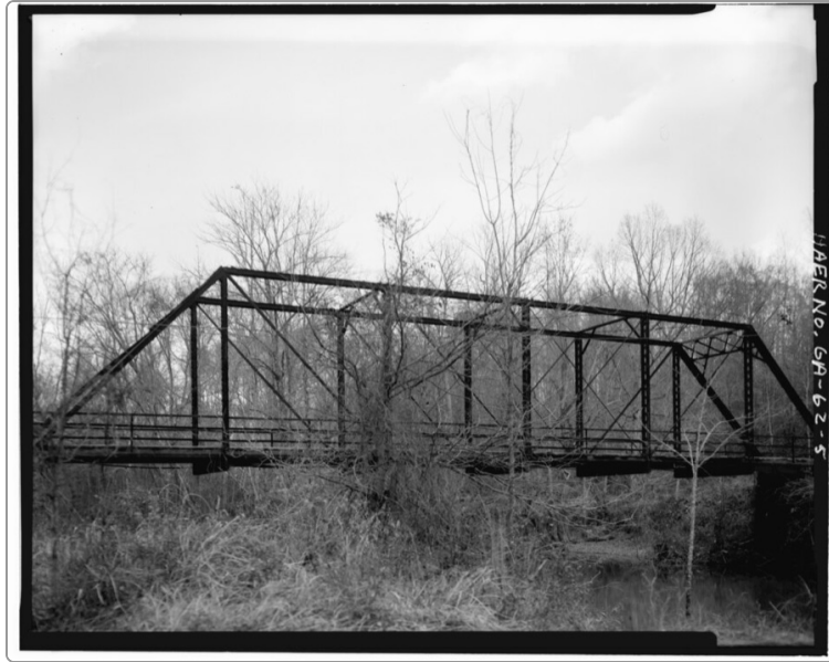
Alcovy Road Bridge: A Pratt Through Truss , Historic American Engineering Record, Photograph of a bridge built in the early 1900s · Photograph · Library of Congress, Prints and Photographs Division
