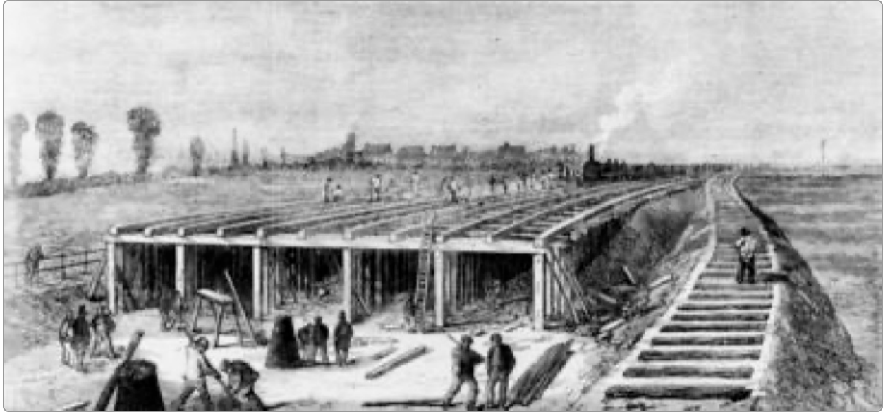
The Northern Outfall Sewer Under Construction , Unknown engraver, about 1859–1865 · Engraving · London
