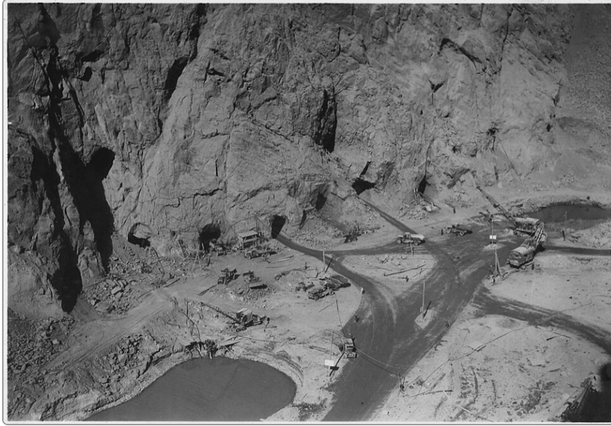
Excavating the Nevada Powerhouse at Hoover Dam, U.S. Bureau of Reclamation, 1932 · Photograph · National Archives and Records Administration
