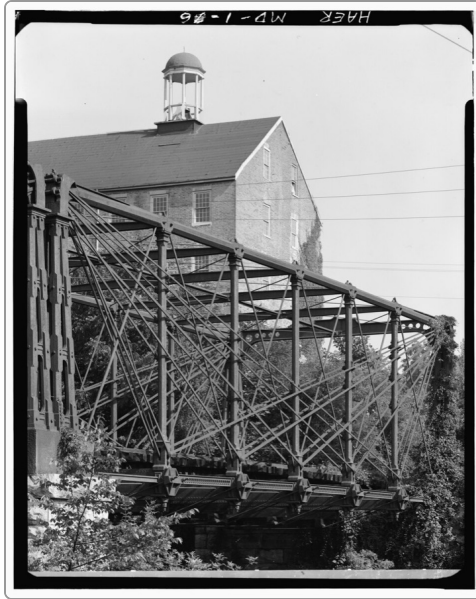
The Bollman Truss Bridge at Savage, Maryland , William E. Barrett, Historic American Engineering Record, 1970 (bridge built 1869) · Photograph · Library of Congress, Prints and Photographs Division Image: Wikimedia Commons , public domain
