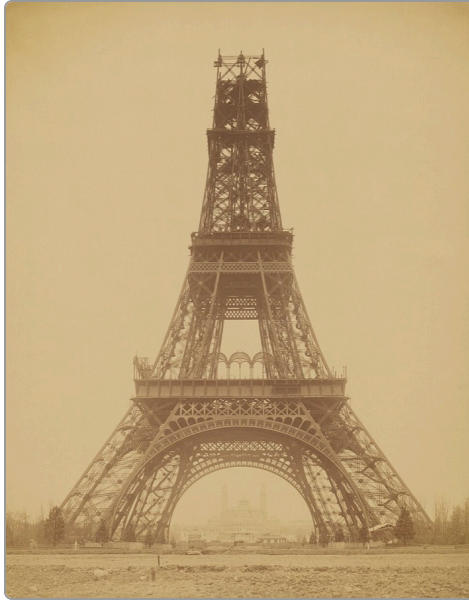
The Eiffel Tower under Construction , Louis-Émile Durandelle, November 23, 1888 · Albumen photograph · From Durandelle's photographs of the tower's construction
