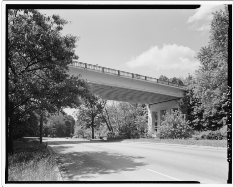
The Walnut Lane Bridge, Philadelphia , Historic American Engineering Record, photograph made for the HAER survey · Photograph · Library of Congress
