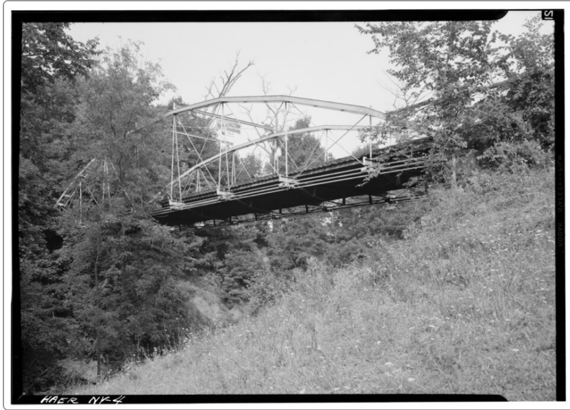
Whipple Bowstring Truss Bridge , Historic American Engineering Record, survey photograph of an 1867 bridge · Photograph · Library of Congress Image: Wikimedia Commons , public domain
