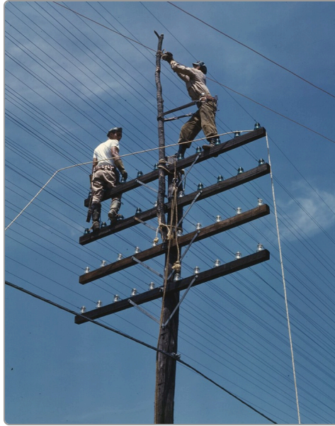
TVA Linemen at Work , Tennessee Valley Authority photographer, 1940s · Color photograph · Tennessee Valley Authority
