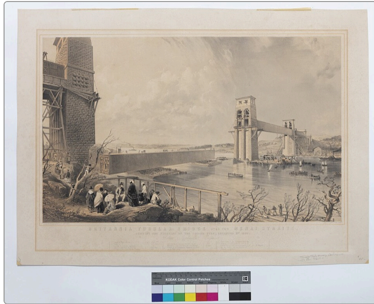
Floating a Tube of the Britannia Bridge , George Hawkins, 1849–1850 · Lithograph · Published in Great Britain; digital copy from the Digital Public Library of America
