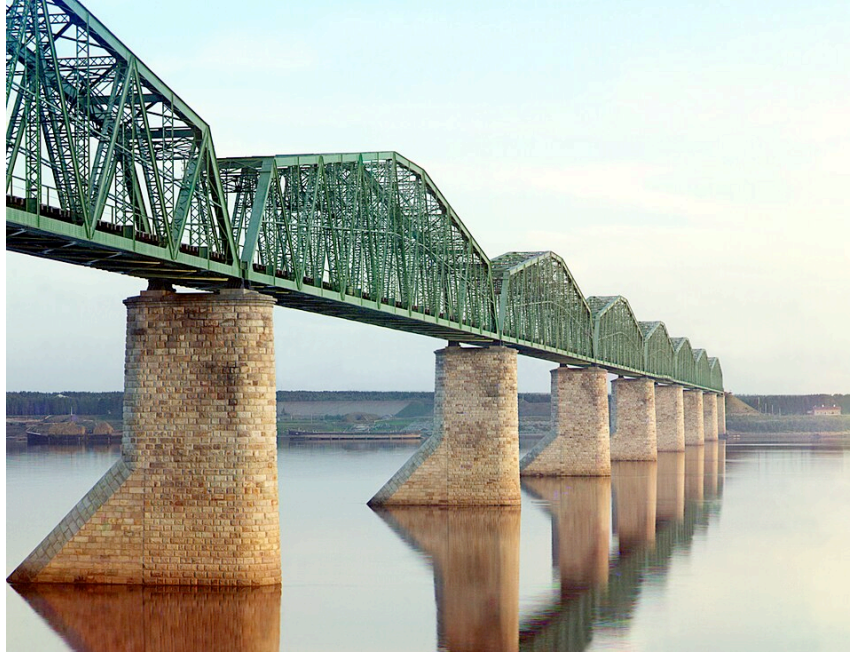
Trans-Siberian Railway Metal Truss Bridge on Stone Piers, over the Kama River near Perm, Ural Mountains Region, Sergei Mikhailovich Prokudin-Gorskii, about 1910 · Color photograph made from a glass plate with three exposures (red, green and blue filters); modern digital color composite · Library of Congress, Prints and Photographs Division, Prokudin-Gorskii Collection, Washington, D.C.
