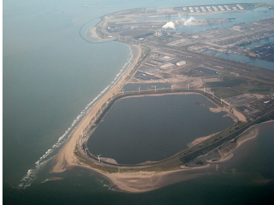
Aerial photograph of the Port of Rotterdam and the Maasvlakte , Photograph by Nitot (Wikimedia Commons), CC BY-SA 3.0, 2007 · Color aerial photograph · Wikimedia Commons
