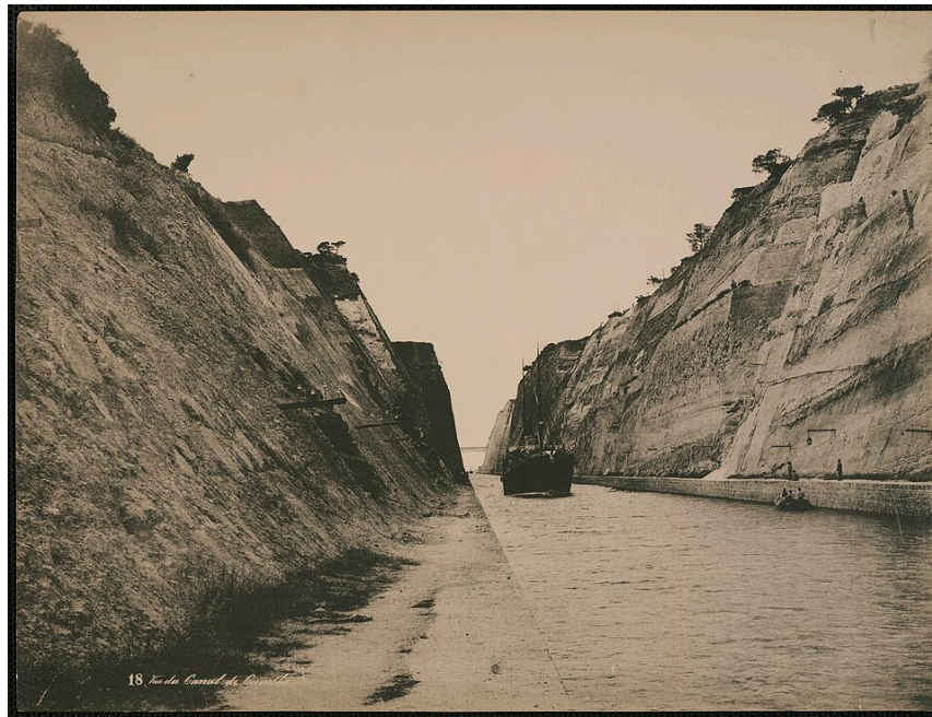
Vue du Canal de Corinthe (View of the Corinth Canal) , Unknown photographer, about 1893–1910 · Collotype print from a photograph · Boston Public Library, Arts Department (Nicholas Catsimpooulas Collection), via Digital Commonwealth; image on Wikimedia Commons
