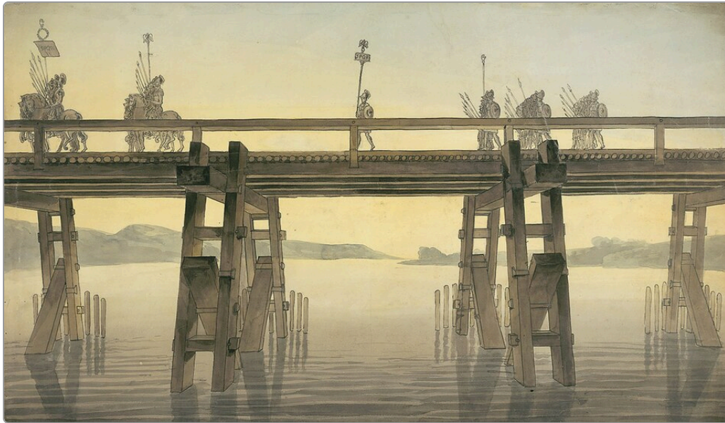
Caesar's Bridge over the Rhine , A reconstruction drawing after Caesar's own description, 19th century · Engraving (reconstruction of the timber bridge of 55 B.C.) · After Julius Caesar, Gallic War , Book 4 Image: Wikimedia Commons , public domain
