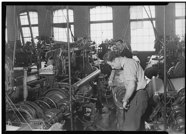
Setting a New Warp onto a Loom, Madison Silk Company, Paterson, Photographer for the Works Progress Administration's National Research Project, c. 1937 · Photograph · U.S. National Archives Image: Wikimedia Commons , public domain
