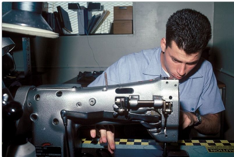
Navy Parachute Rigger Threading an Industrial Sewing Machine, U.S. Navy photographer, Mid-20th century · Photograph · U.S. National Archives (via the Digital Public Library of America)
