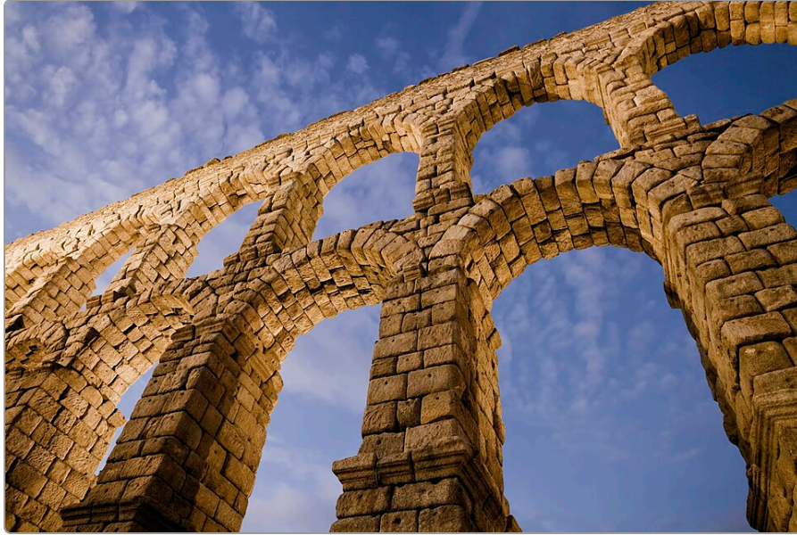
The Aqueduct of Segovia , Roman builders (photograph by David Corral Gadea), c. A.D. 100 · Granite blocks, laid without mortar · Segovia, Spain
