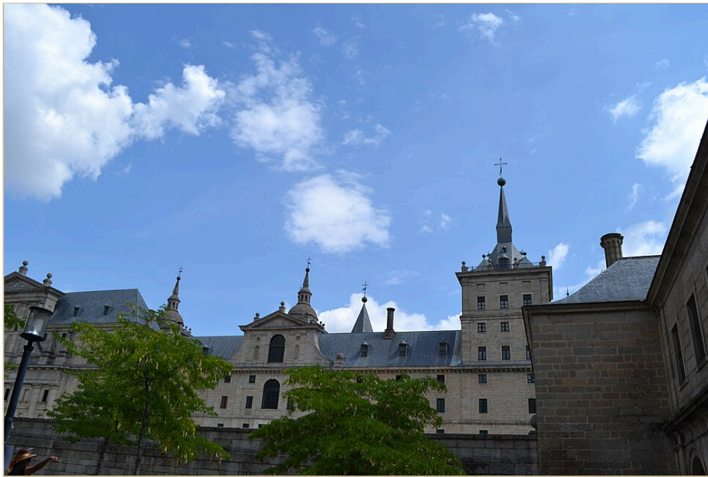
The Monastery of El Escorial , Juan Bautista de Toledo and Juan de Herrera, architects (photograph by Dorieo), 1563–1584 · Granite, with slate roofs · San Lorenzo de El Escorial, near Madrid, Spain
